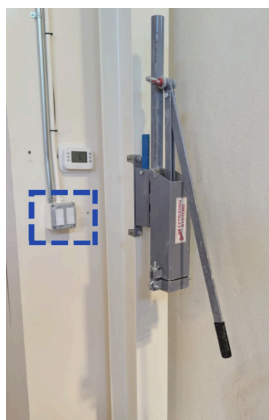
TUNNEL BY EXTRUDER
